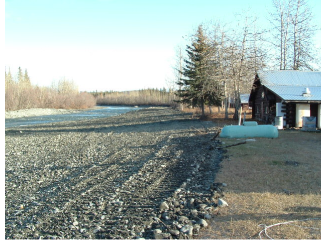
Photo 2: After erosion protection has been installed, looking east adjacent to Gakona Lodge, October 2004.
