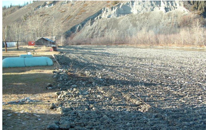
Photo 3: After erosion protection has been installed, looking west adjacent to Gakona Lodge, October 2004.
