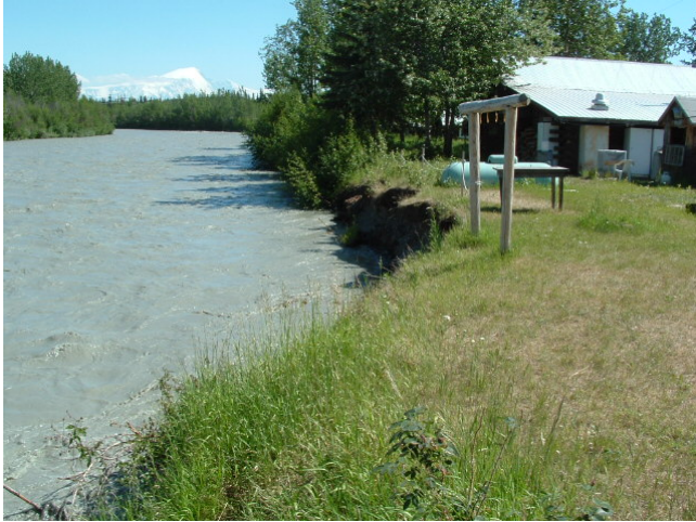
Photo 1: Erosion, looking east adjacent to the Gakona Lodge, July 2004.
